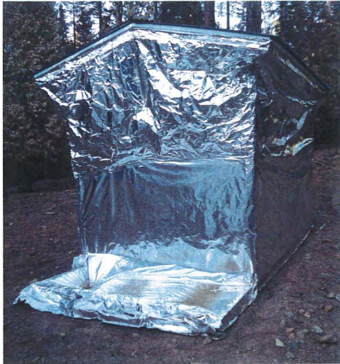
Photo 1; Wellhouse with Fire Resistant Foil
