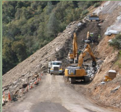
Spring 2015 Phase I remove talus (30,000 CY removed)
