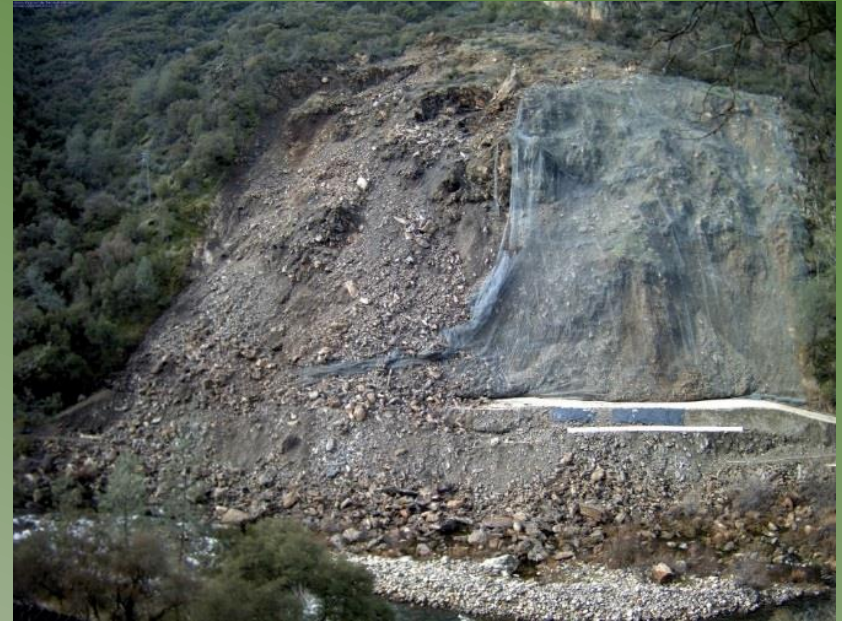
Photo: Discovery in the morning after the November 2015 slide event taking down cable net drapery.
